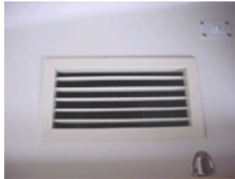
Air Conditioning Vent in Main Salon
