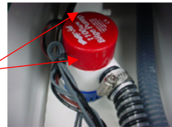
Forward Bilge Pump with Float Switch
