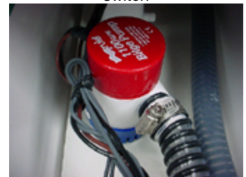
Forward bilge pump with float switch
