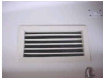
Air conditioning vent In main salon
