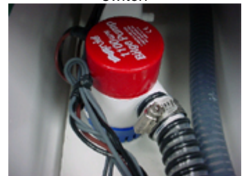
Forward bilge pump with float switch
