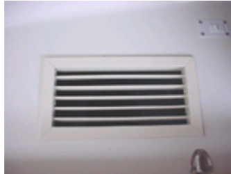
Air conditioning vent In main salon
