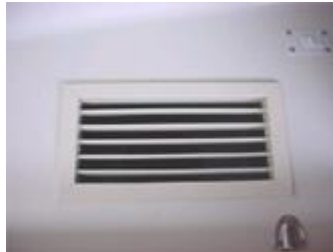
Air conditioning vent In main salon
