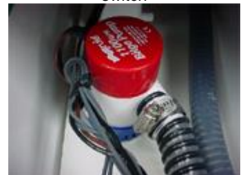
Forward bilge pump with float switch
