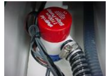
Forward bilge pump with float switch
