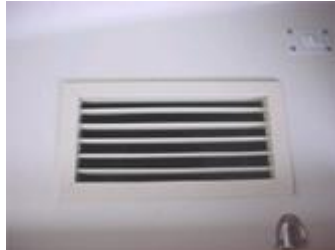
Air conditioning vent in main salon
