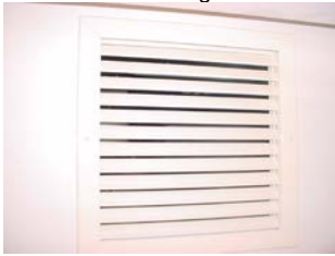
Air Conditioner Return on the face of the V Berth storage area
