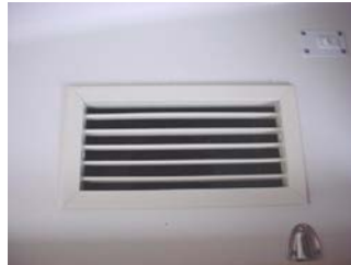
Air Conditioning Vent in Main Salon
