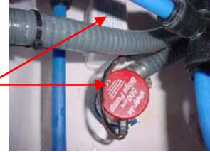
Forward Bilge Pump with Float Switch
