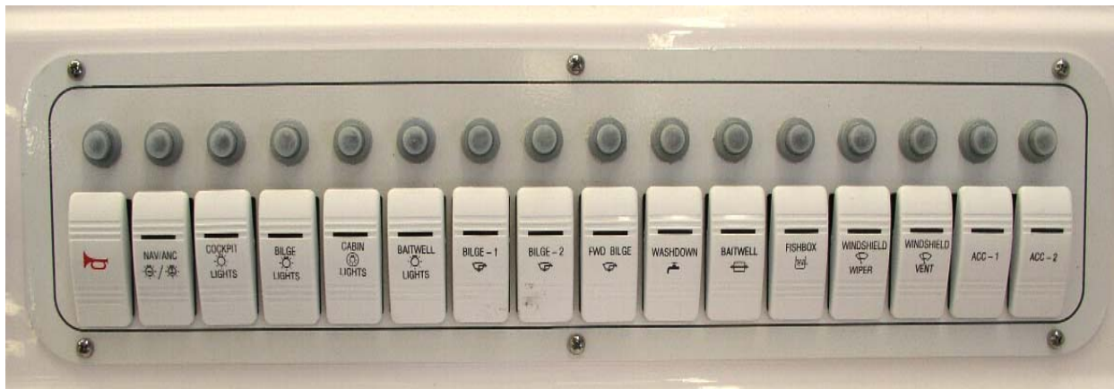
Circuit Breakers – On the switch panel above the individual switches
