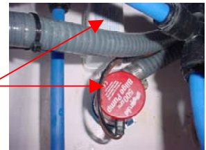
Forward Bilge Pump with Float Switch
