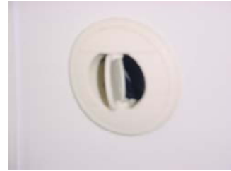
Air Conditioning Vents in Mid Berth Cabin and Head
