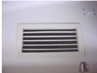
Air Conditioning Vent in Main Salon
