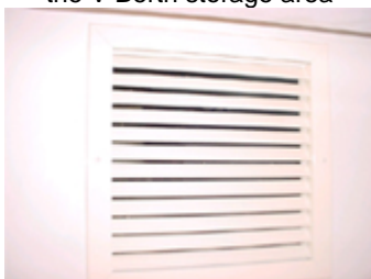
Air Conditioner Return on the face of the V Berth storage area
