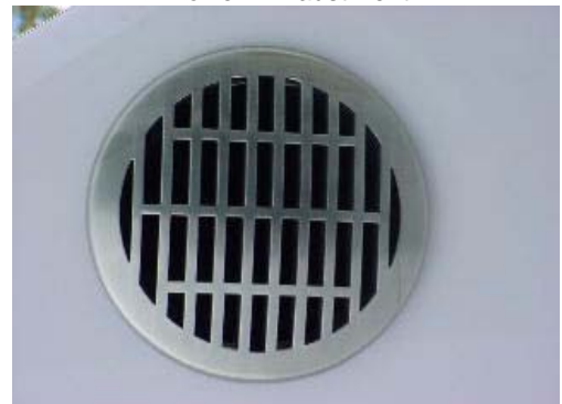
Blower Exhaust Vent
