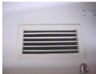
Air Conditioning Vent in the Main Salon
