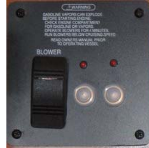
Blower Switch – Next to the AC/DC Panel
