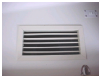
Air Conditioning Vent in the Main Salon
