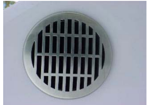
Blower Exhaust Vent
