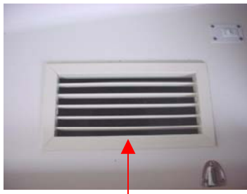
Air Conditioning Vent in the Main Salon
